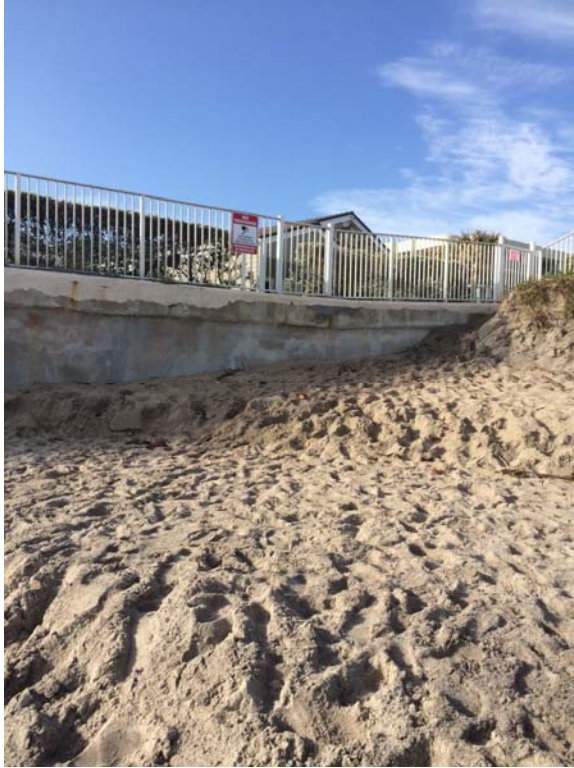
Western end of return, good condition:
