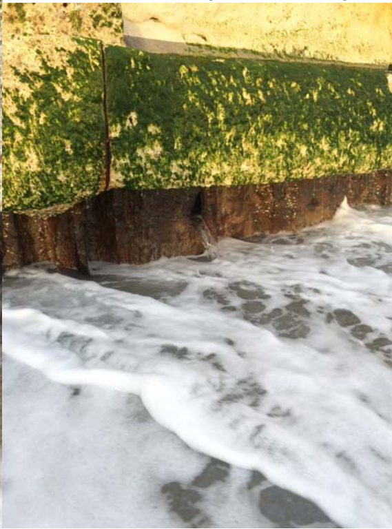
Substantial loss of backfill thru toewall hole:
