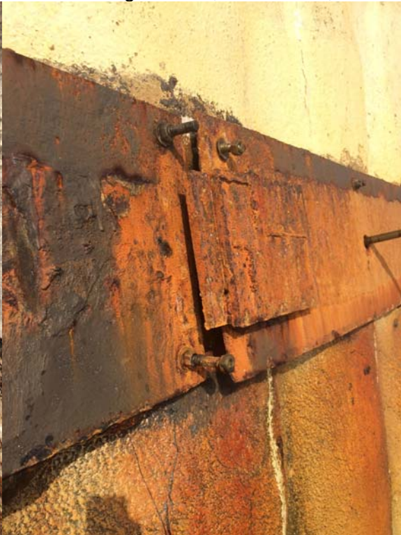
Severe rusting of waler; loss of nuts, washers:
