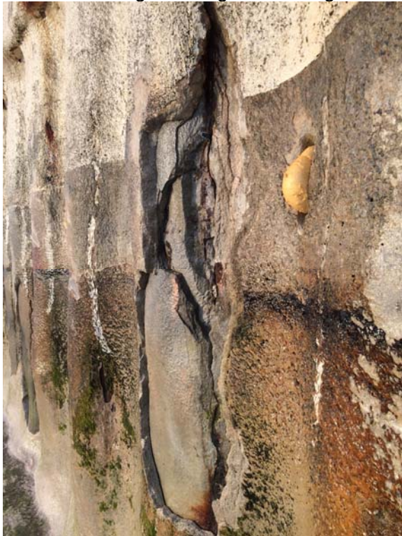
Concrete facing cracking and rusting:
