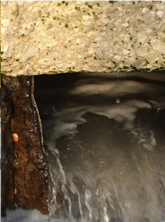
Substantial loss of backfill thru toewall hole:
