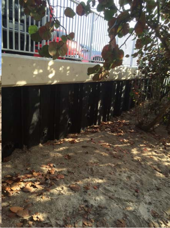
Parking lot seawall, good condition:
