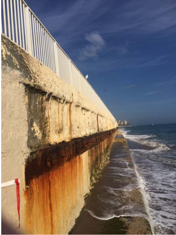
Concrete facing cracking and rusting:
