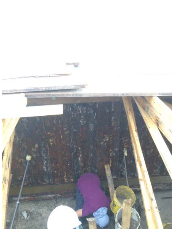
Severe rusting of waler; loss of nuts, washers:
